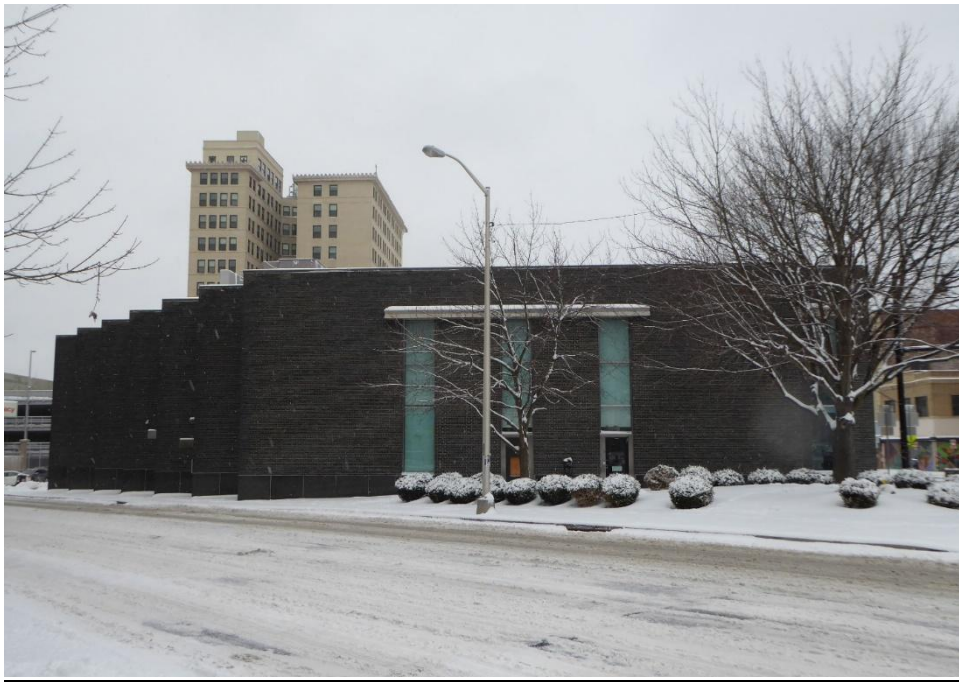
Figure 3: Mellon National Bank, East Liberty Office, showing southeast (side) facade, facing northwest (Mary Barenfeld).
