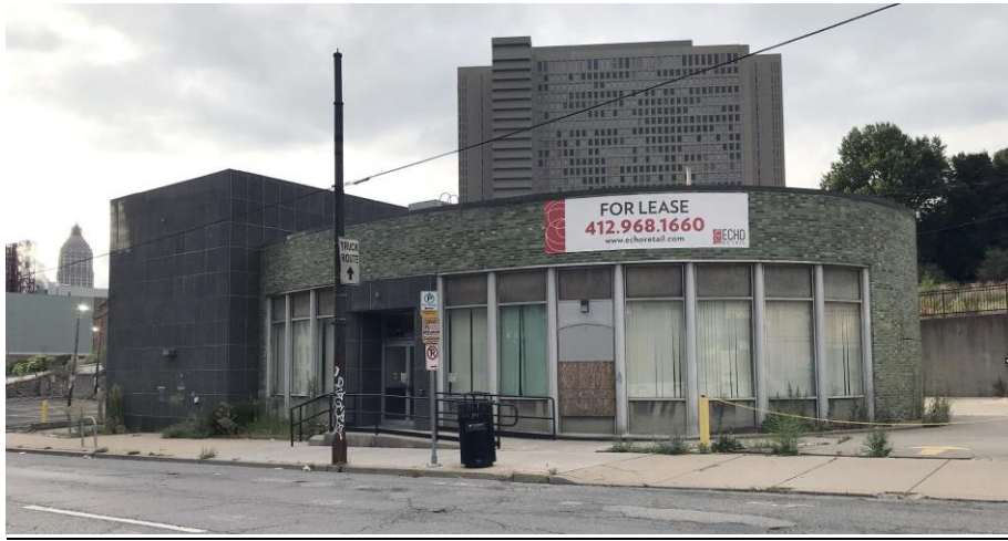
Figure 8: Upper Fifth branch. Location: 1425 Fifth Avenue, Pittsburgh PA 15219. Current Use: Vacant. Source: Brittany Reilly, August 2020.
