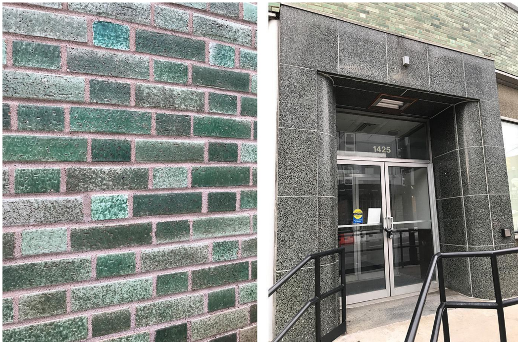
Figure 9: Upper Fifth branch. Material and details match 6112 Penn Ave. Location: 1425 Fifth Avenue, Pittsburgh PA 15219. Current Use: Vacant. Source: Brittany Reilly, August 2020.
