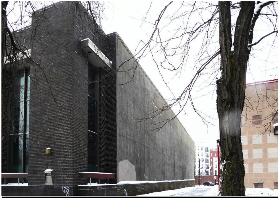
Figure 6: Mellon National Bank, East Liberty Office, showing northwest (side) facade, facing south (Mary Barenfeld).
