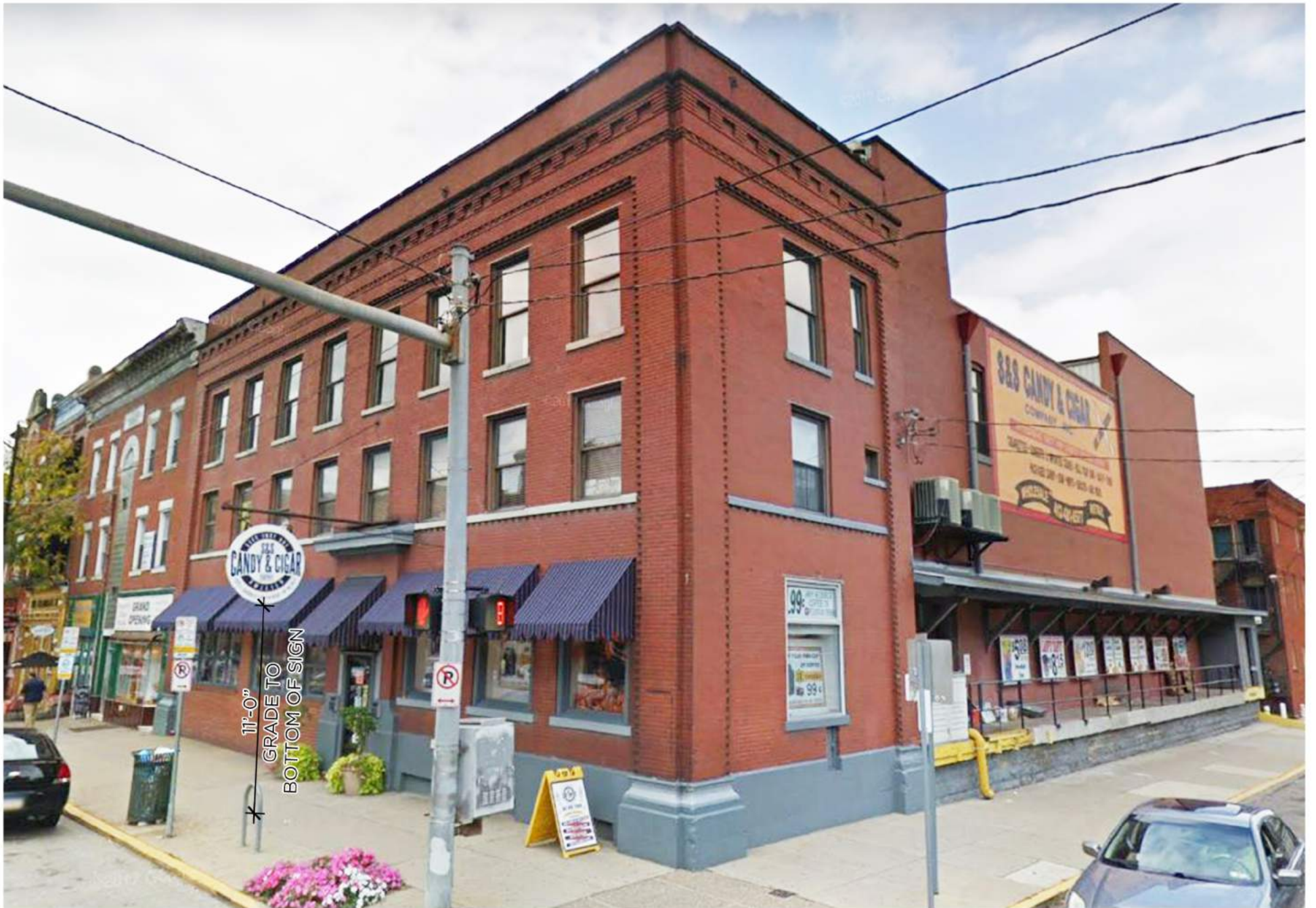
REPLACE NONCONFORMING SIGN WITH NEON SIGN TO MATCH. EXISTING SUPPORT TO REMAIN.
