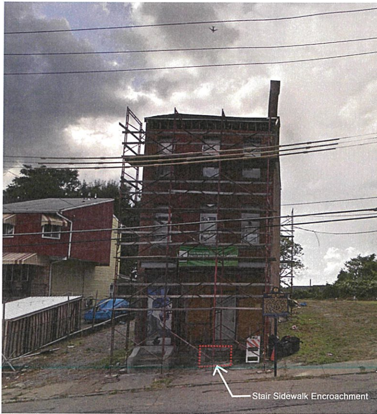
Exterior Photo 1: 1727 Bedford avenue
