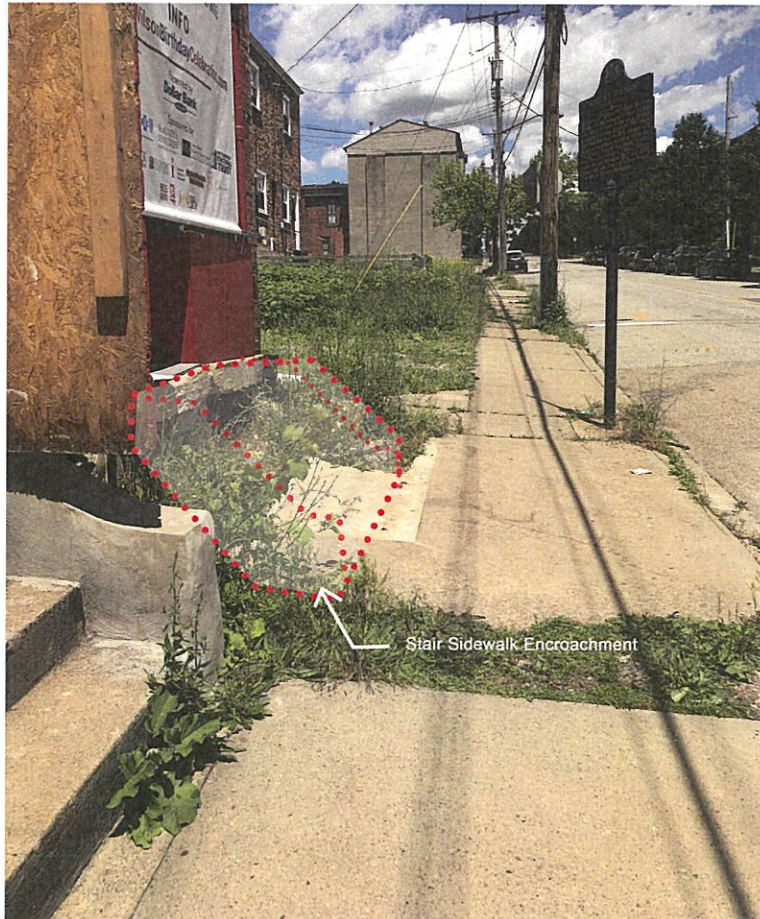
Exterior Photo 2: 1727 Bedford avenue
