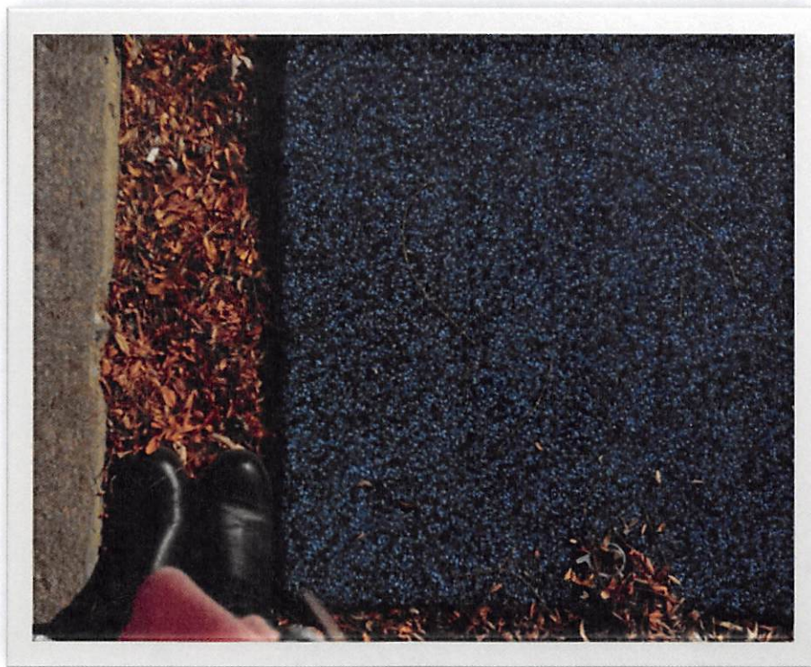
Picture 2: Fairywood Park example of PIP safety floor with shrinkage but in fair condition
