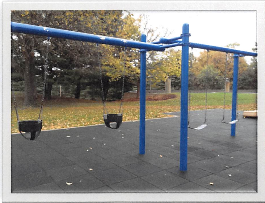
Picture 1: Schenley Park example of rubber tiled safety surface in good condition
