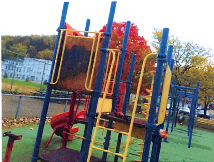
57 th Street Playground - Missing Equipment – Rated Poor
