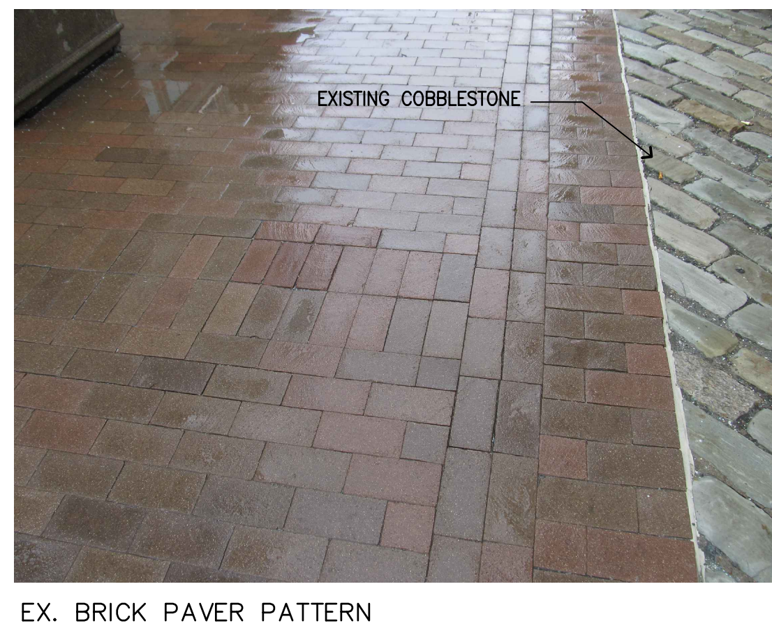
F BRICK PAVERS AT COBBLESTONE PLAZA SCALE: 3/4" = 1'-0"
