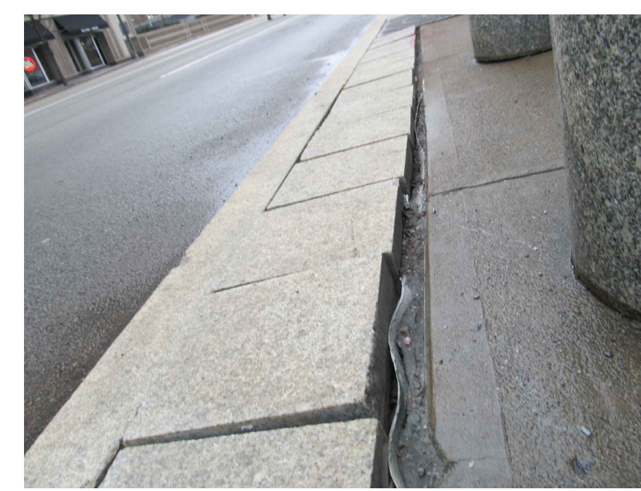
8 GRANITE PAVER STRIP ALONG CURB
