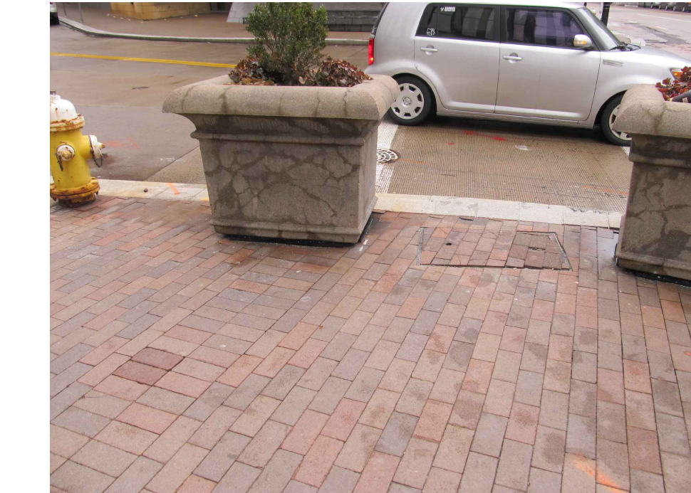
4 TRAFFIC SIGNAL ACCESS PANEL
