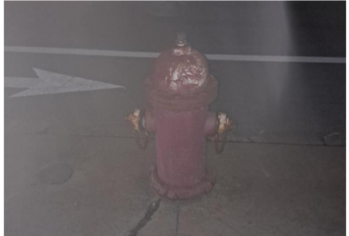
Hydrant C188 (North facing)
