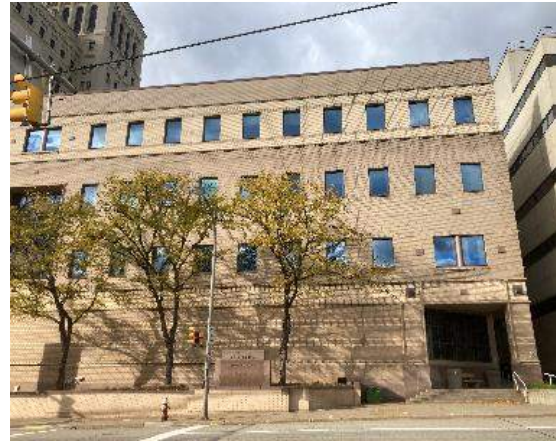
11 East Wing Medical Offices
