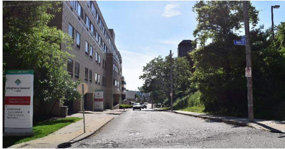
Existing Hemlock St looking west towards Sandusky St
