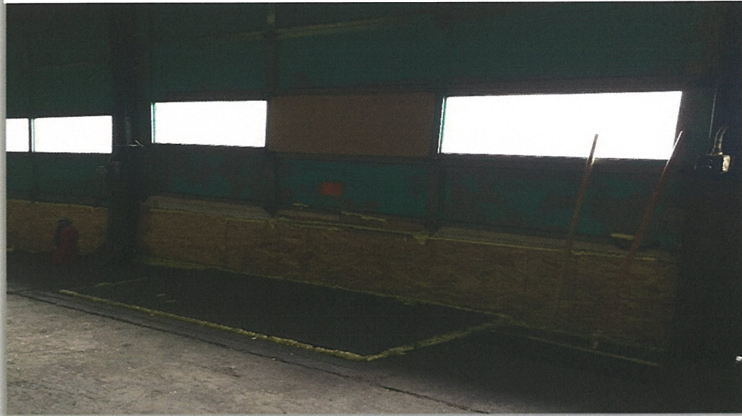
Photo 3 - Interior Bay Door
