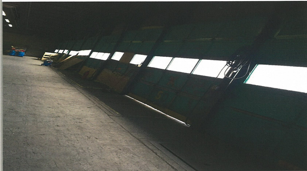
Photo 4 - Interior Bay Doors
