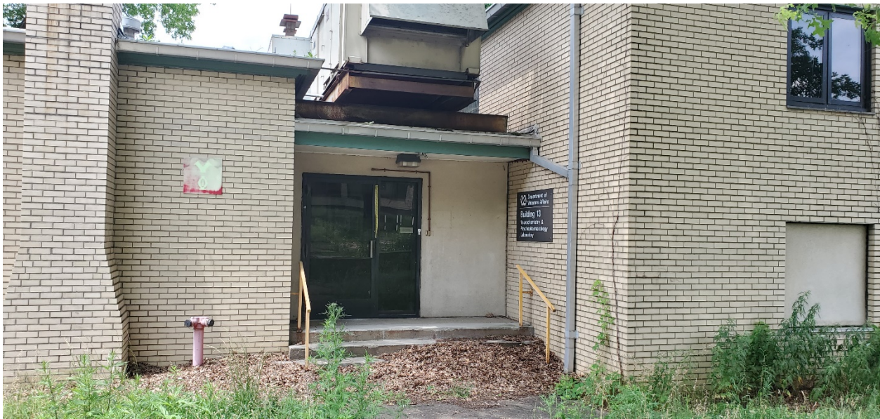
Entry bridge with mechanical system above
