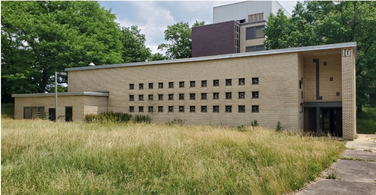
North Façade, slab glass windows
