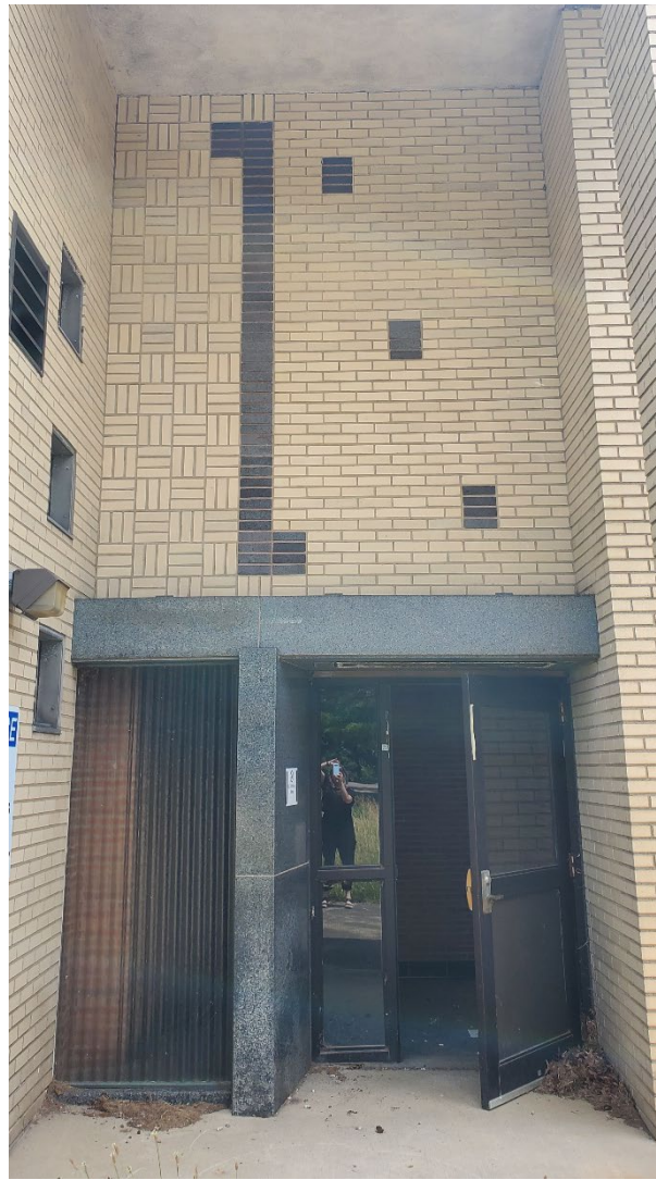
Entry façade decorative elements
