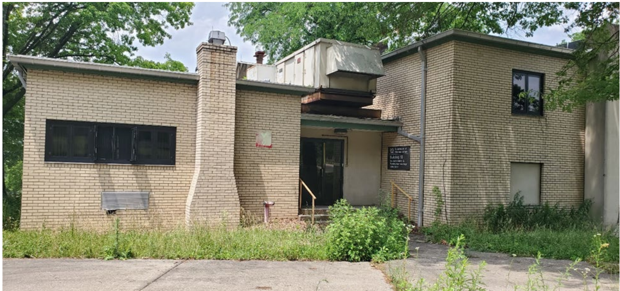
Building 13 East Facade
