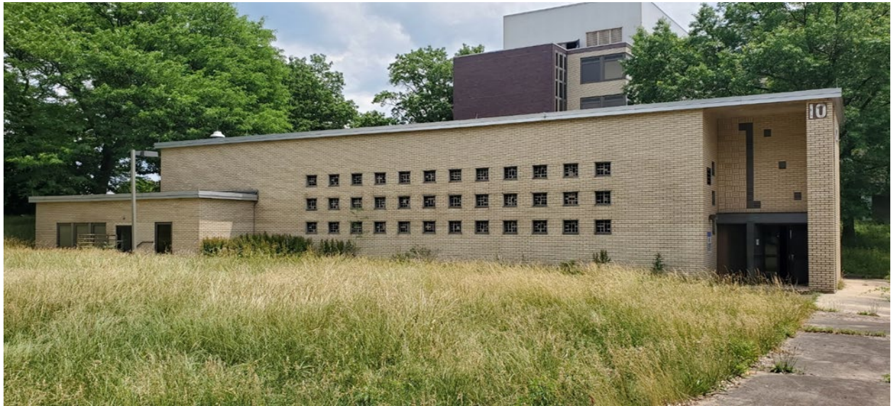
Building 10 North Facade
