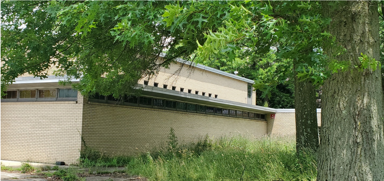
South façade, clerestory windows below overhang, slab glass windows above, door on far right out to overhang
