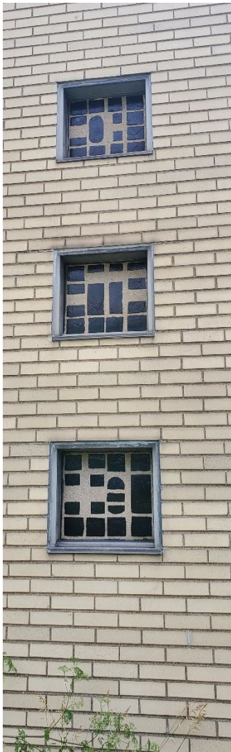
Slab glass detail
