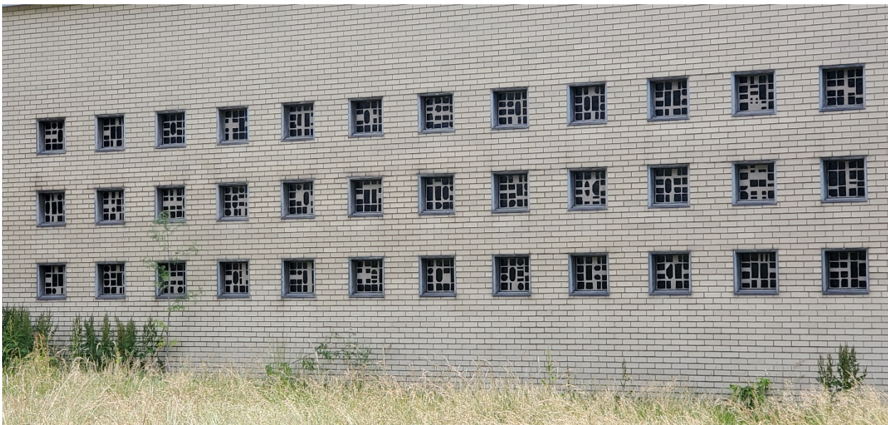
Slab glass, thick pieces of glass inset into concrete
