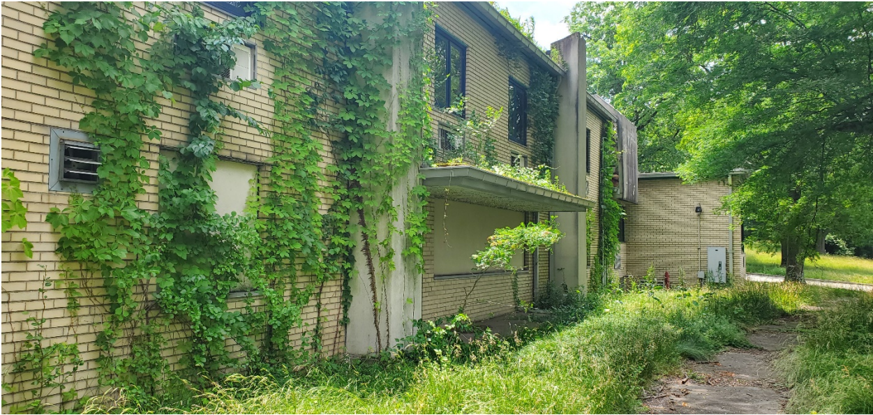
Western elevation looking south, engaged concrete columns and ivy growth
