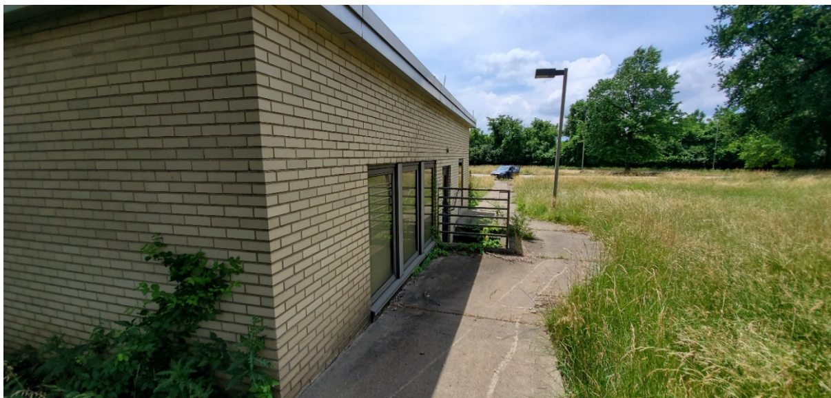
North façade, second entry with stairs
