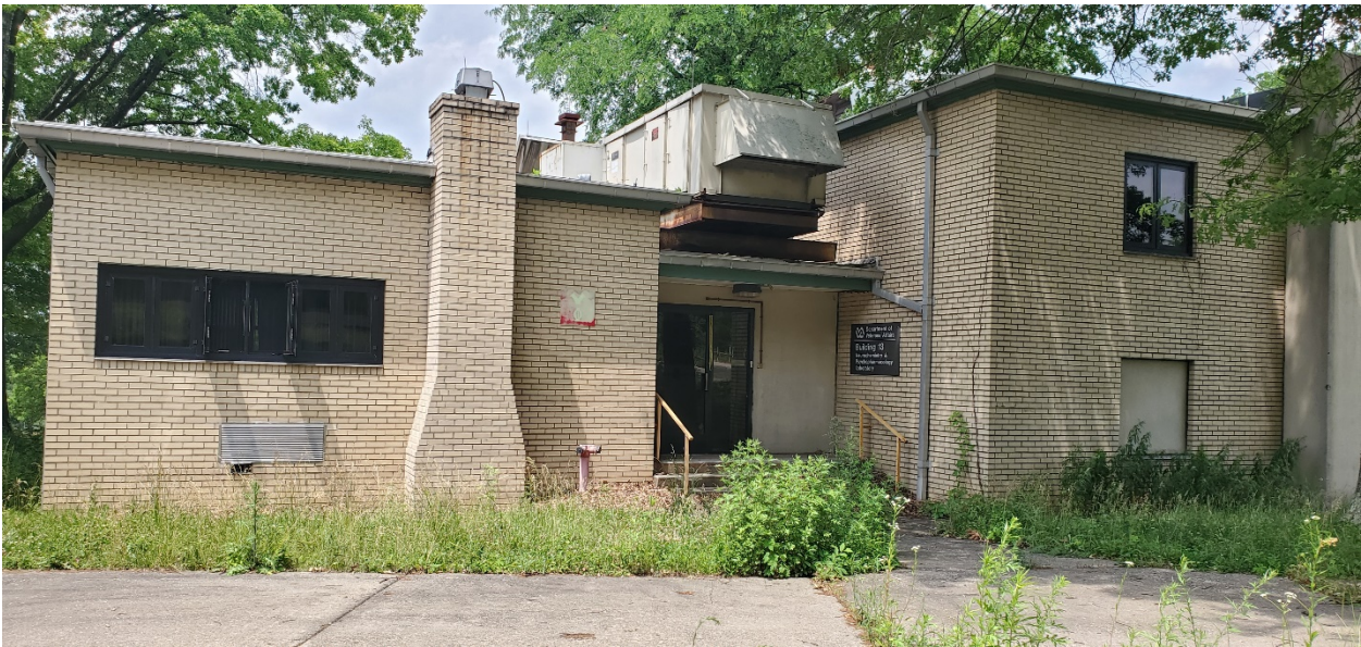
Eastern elevation, one-story south section and middle entry bridge
