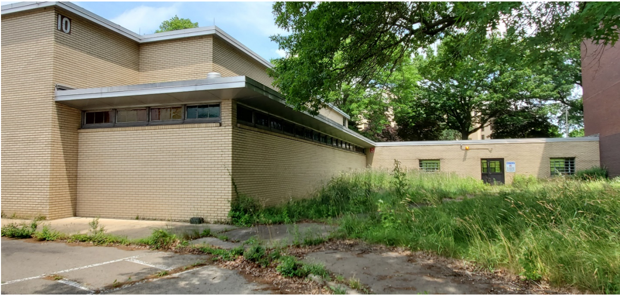
West façade, clerestory windows
