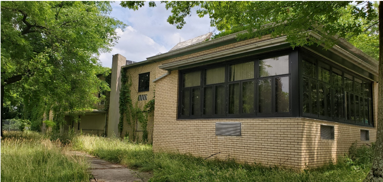
Eastern elevation, one-story south section, with continuous ribbon window
