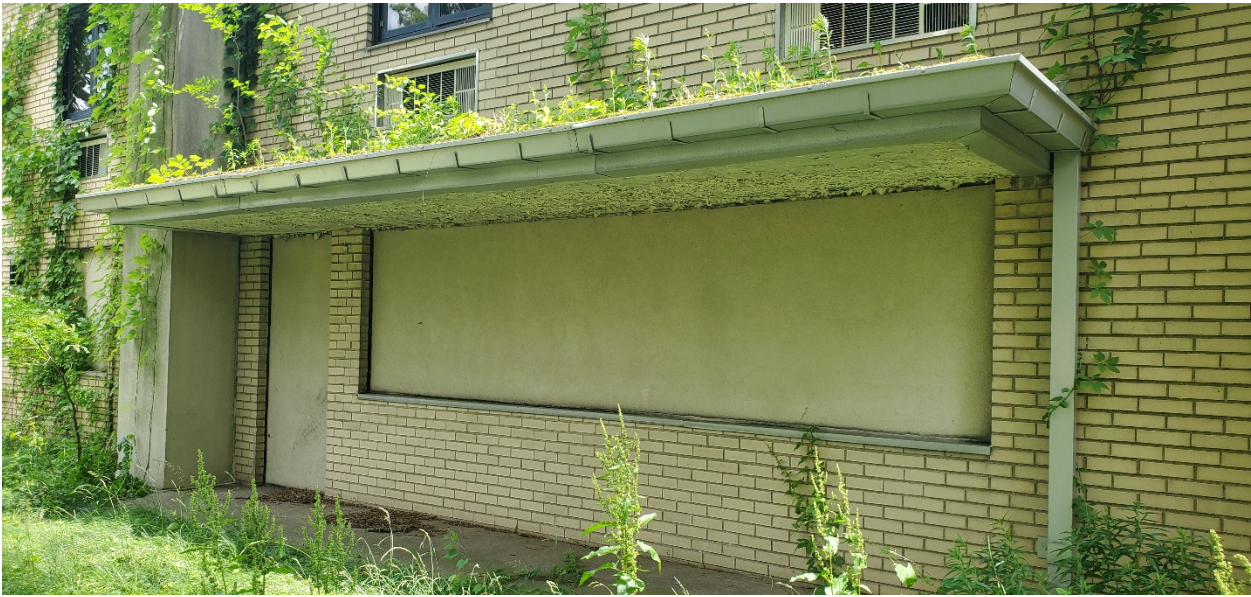
Western elevation entry door, picture window, and overgrown canopy
