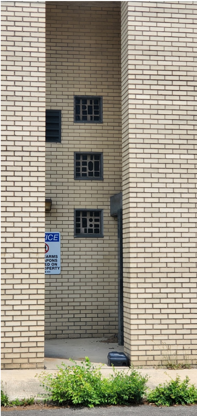
West façade, slab glass detail
