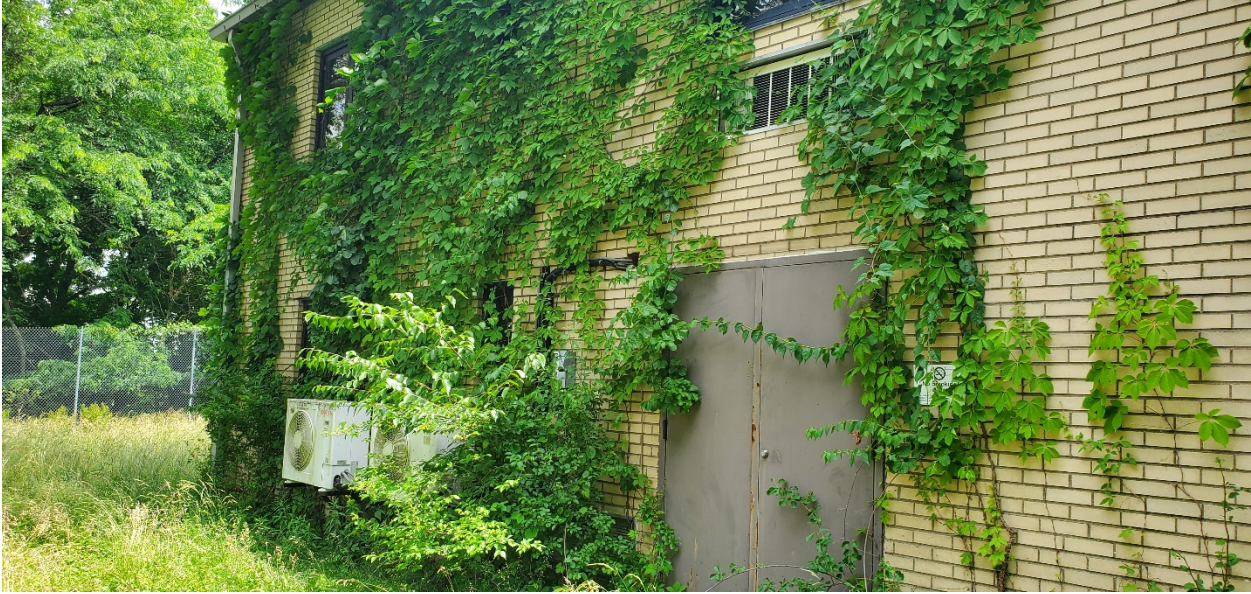
Western elevation, two-story north section, overgrown with ivy
