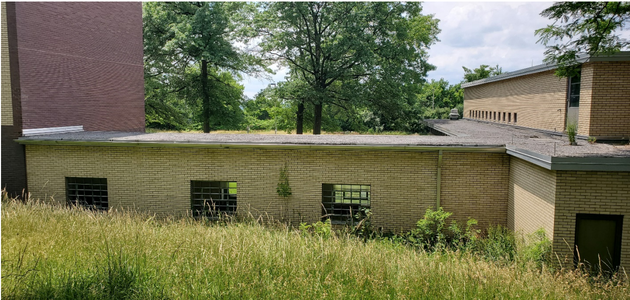
East façade, tunnel fenestration
