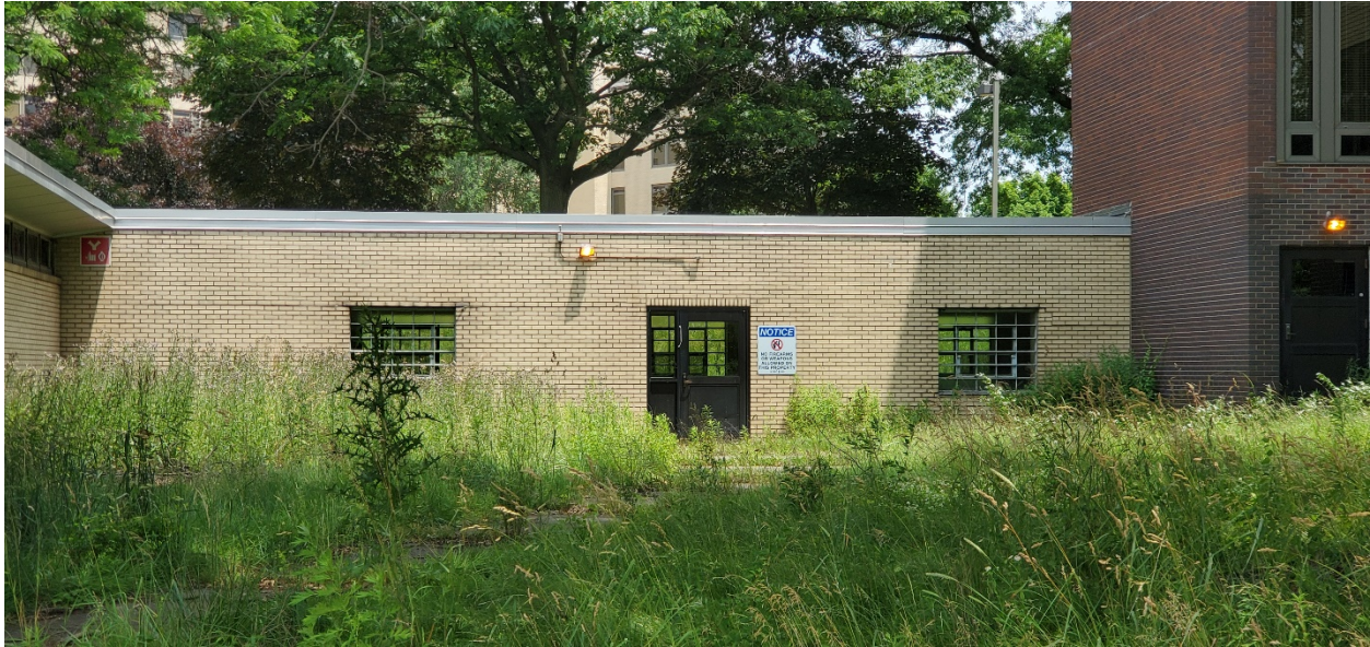
West façade, tunnel
