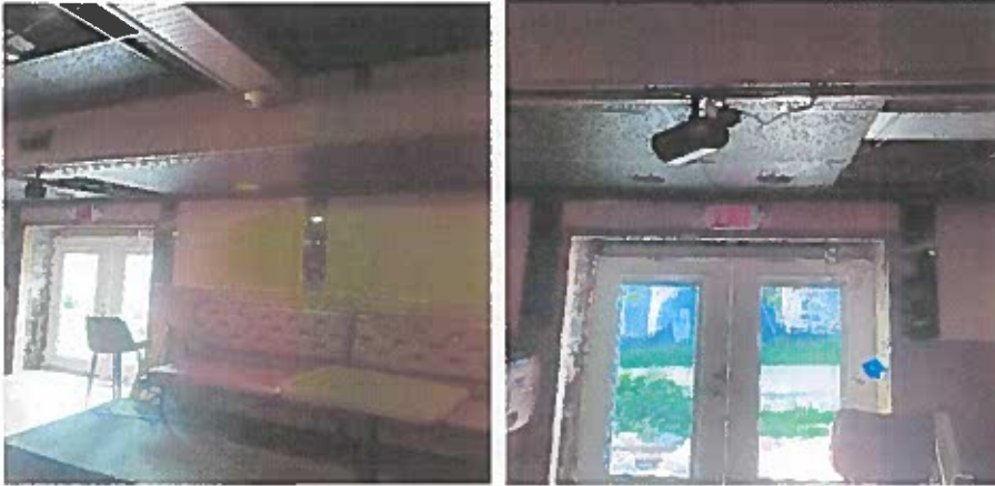
Camera #3 – over main entrance – two views
