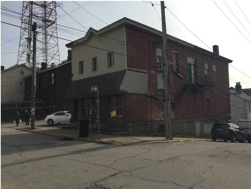
Photo 2: 131 Shiloh – Building front and right side – picture facing east
