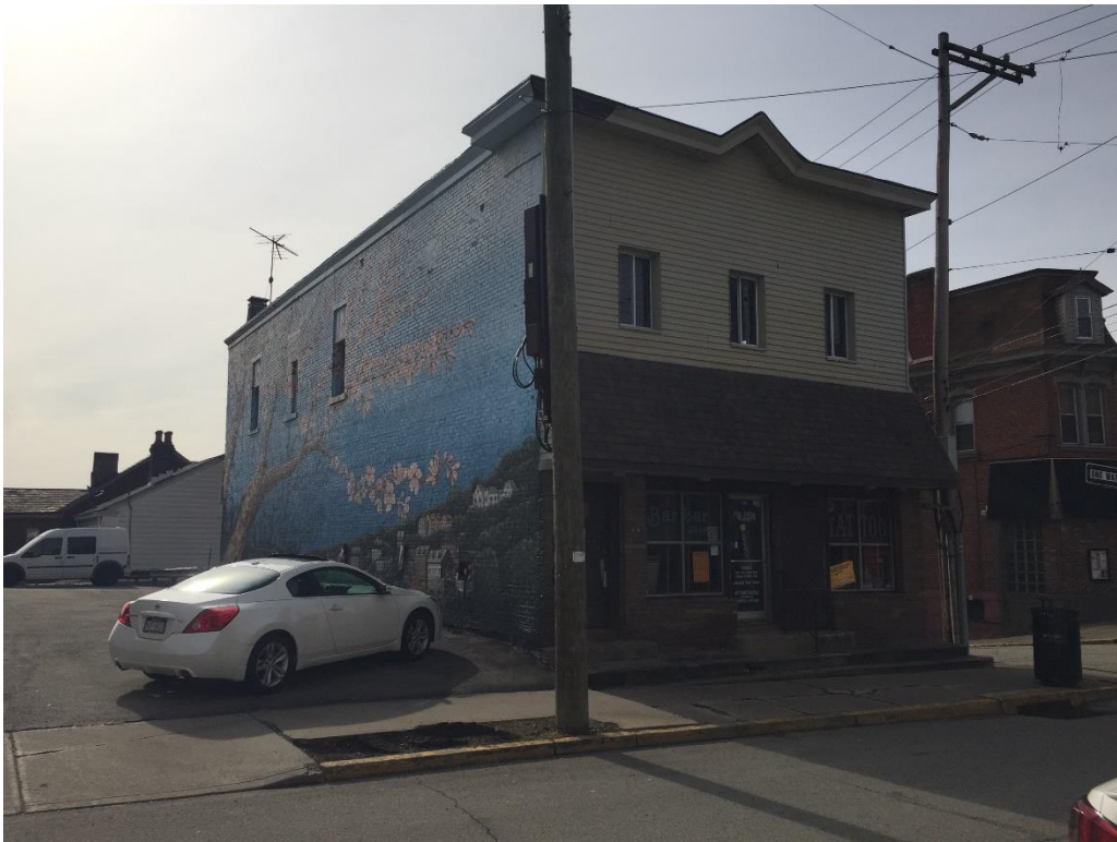
Photo 4: 131 Shiloh – Building front and left side – picture facing south
