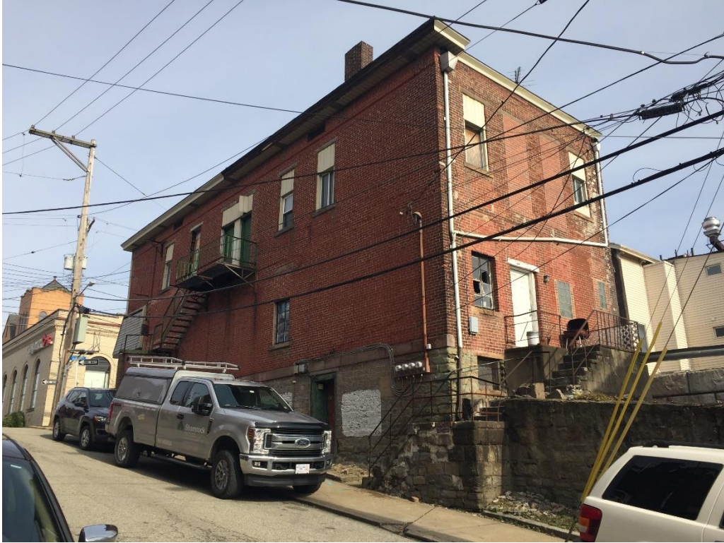
Photo 5: 131 Shiloh – Building rear and right side – picture facing west
