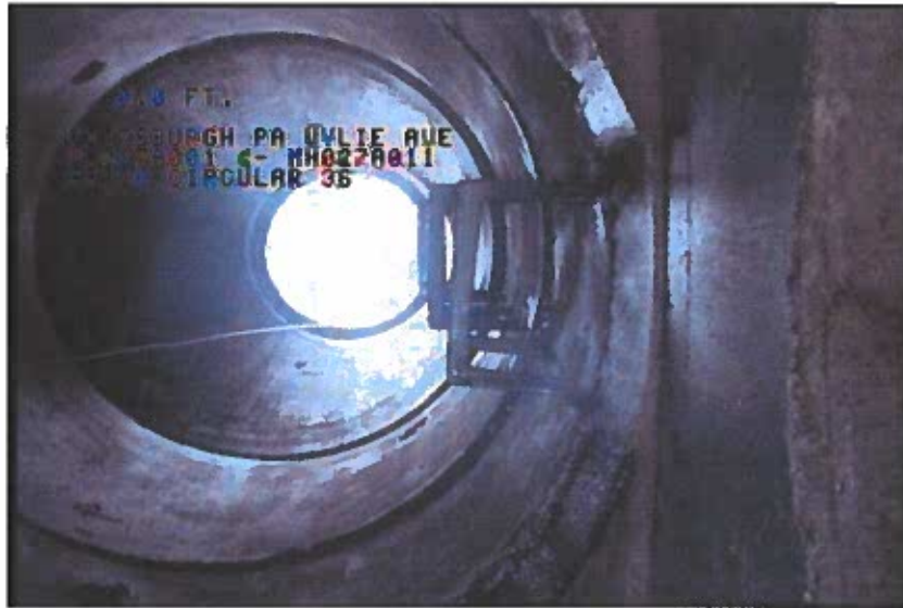
Photo: 3_1A, 00:00:27 0FT, Downstream Manhole, Survey Begins
