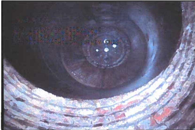
Photo: 3_10A, 00:09:38 153.1FT, Upstream Manhole, Survey Ends
