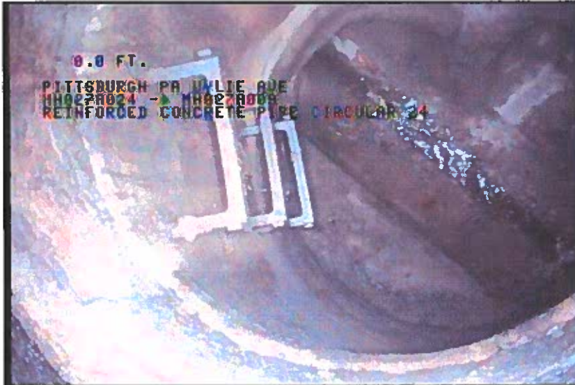
Photo: 2_1A, 00:00:18 0FT, Upstream Manhole, Survey Begins
