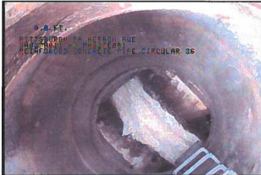
Photo: 1_1A, 00:00:21 0FT, Upstream Manhole, Survey Begins
