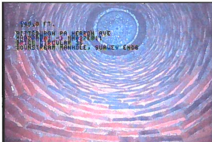
Photo: 1_13A, 00:13:57 149FT, Downstream Manhole, Survey Ends
