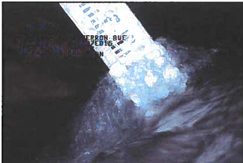
Photo: 4_3A, 00:04:32 0FT, General Observation / FLOW MEASUREMENT 6:12AM
