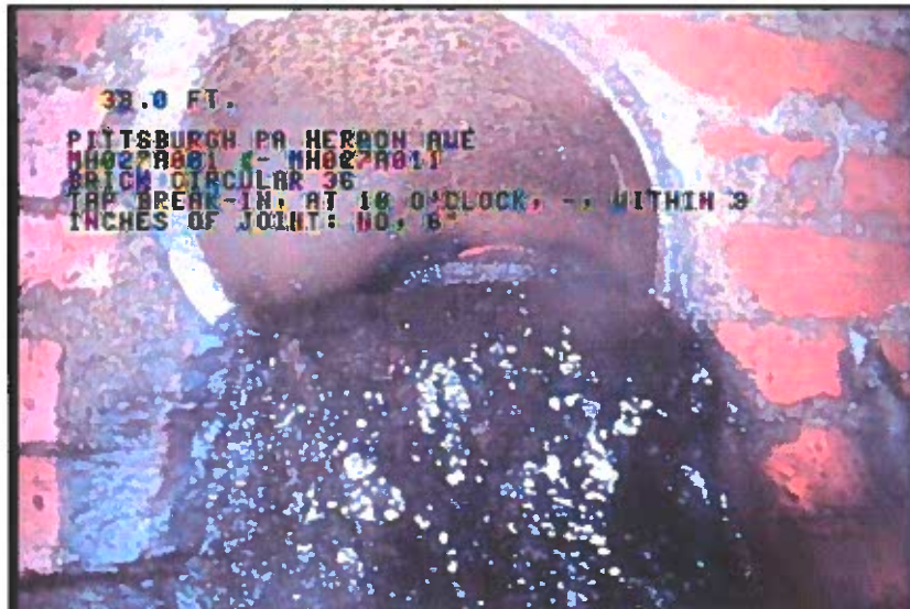
Photo: 3_5A, 00:04:09 38FT, Tap Break-In, at 10 o'clock, -, within 8 inches of joint: NO, 6" / DEPOSITES
