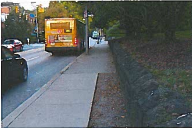
Lack of Buffer at Sidewalks
