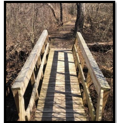
Figure 12: Bridge, Trough Trail
