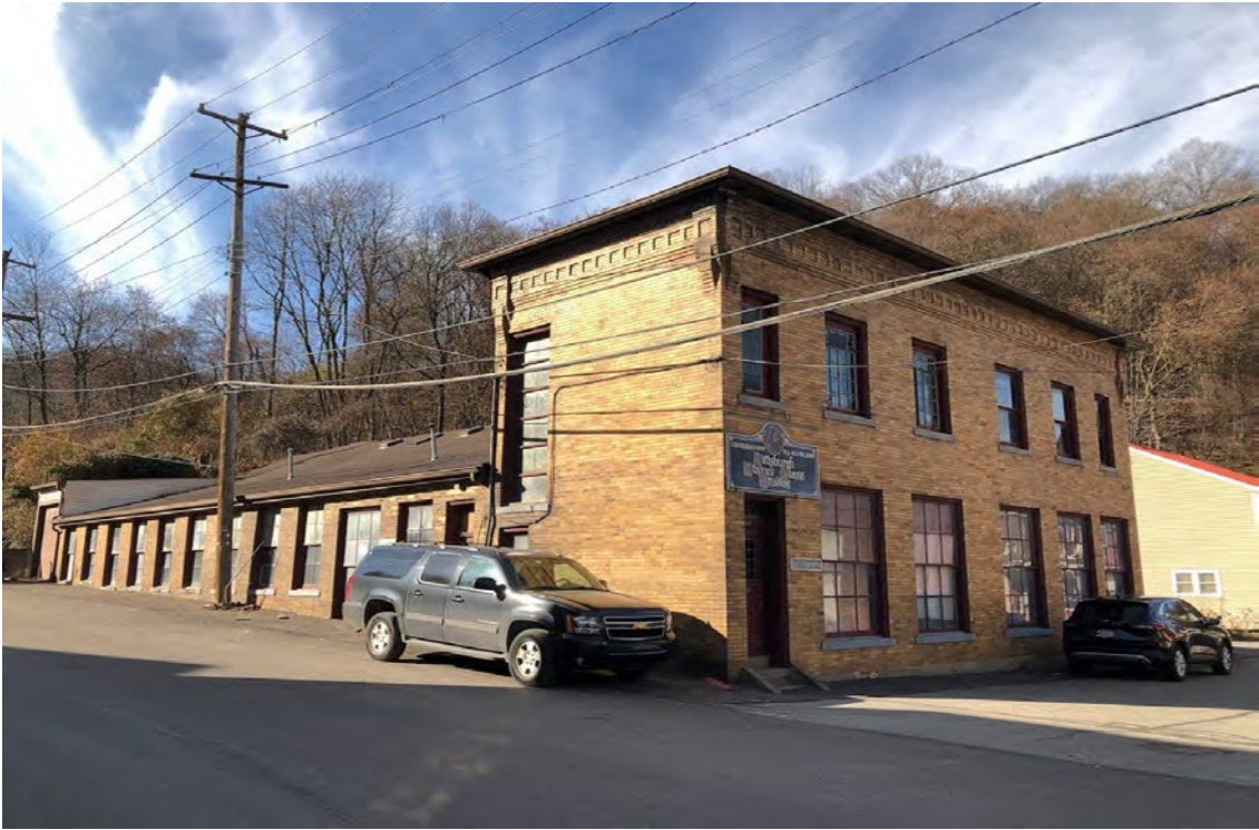
Photo 2. South facade (left) and front facade (right), looking northwest, showing the early-twentieth century “headhouse and shed” design.
