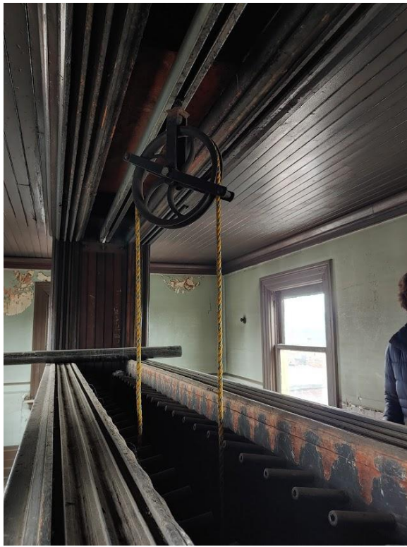
Photograph 5. Pittsburgh EMS Station, Hose Tower, Interior. Source: Dana Cress.
