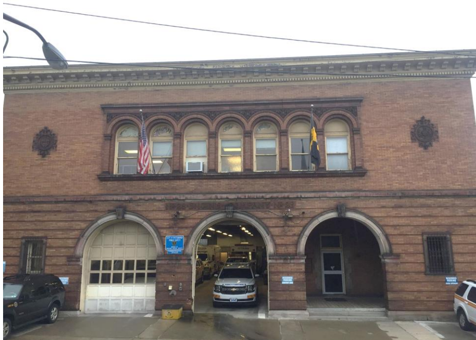
Photograph 2. Pittsburgh EMS Station, Filbert Street Facade, Facing Southwest. Source: Calvin A Yoder.
