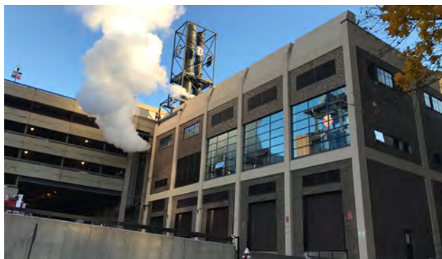
View of the Cogeneration Plant
