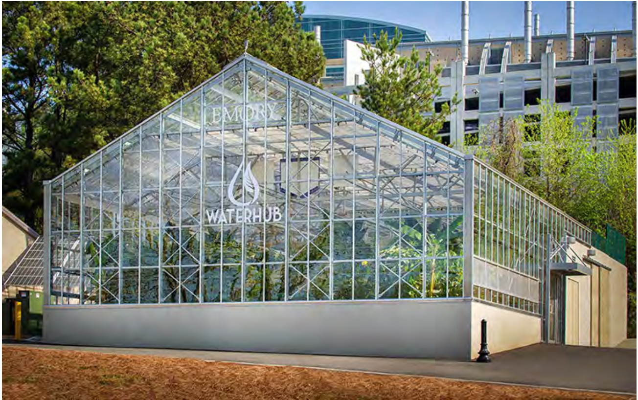
Similar facility at Emory University to proposed WaterHub® wastewater reclamation and reuse system
