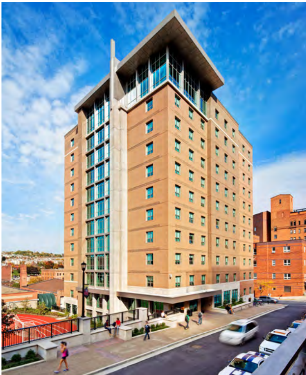
The most recent residence hall, Des Places, achieved a sustainability rating of LEED Gold
