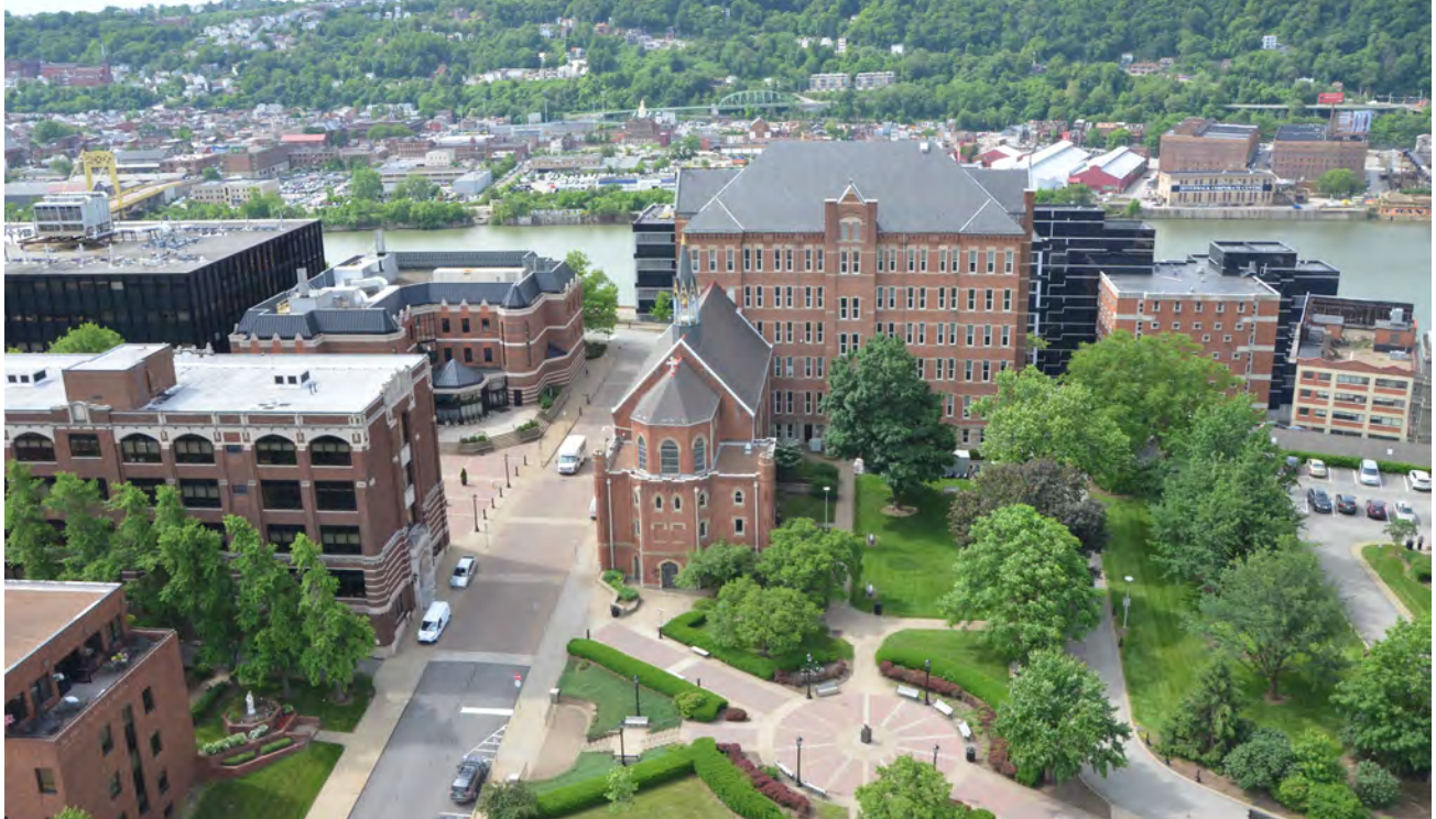
Aerial view from Trinity Green over Administration Building toward the Monongahela River and the Southside Slopes
