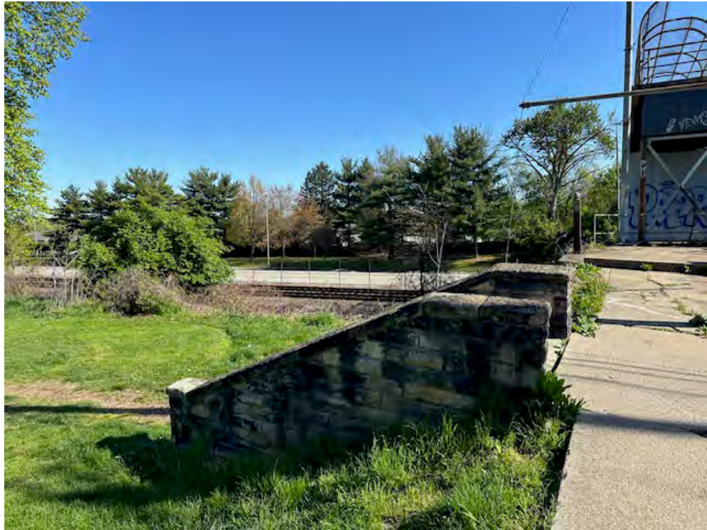
Photo 9. Westinghouse Park, Stone Stairs looking North.
