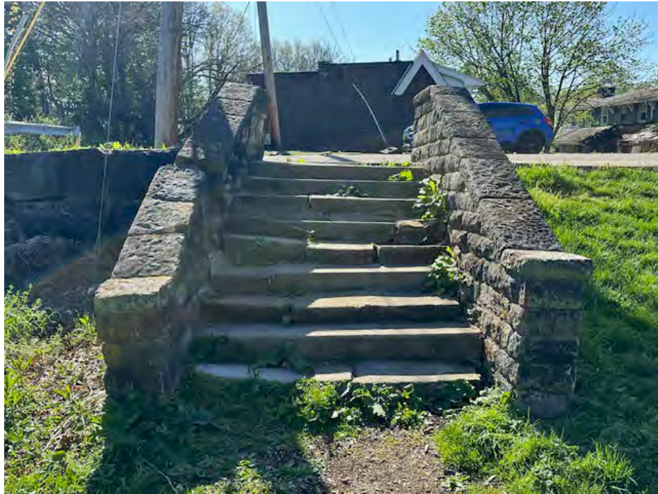
Photo 11. Westinghouse Park, Stairway looking Southeast.
