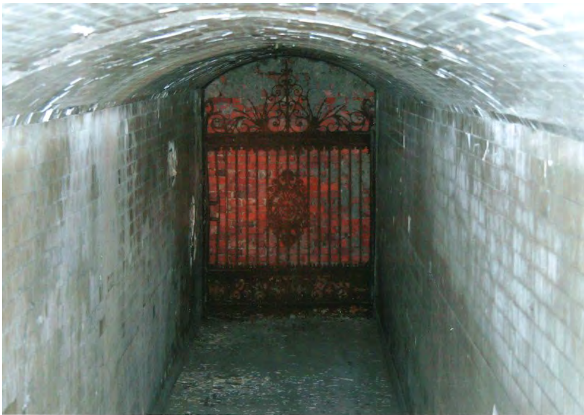
Archeological Photo 9: Lang Avenue tunnel iron gate
