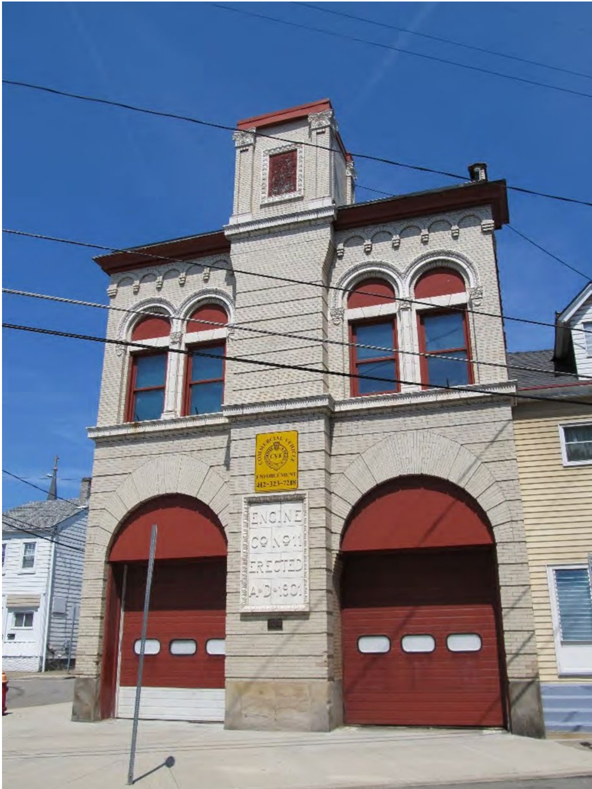
Photo 1: 1800 Ley Street, Troy Hill Fire House, Facing Northwest. Amanda Stander, 2020.
