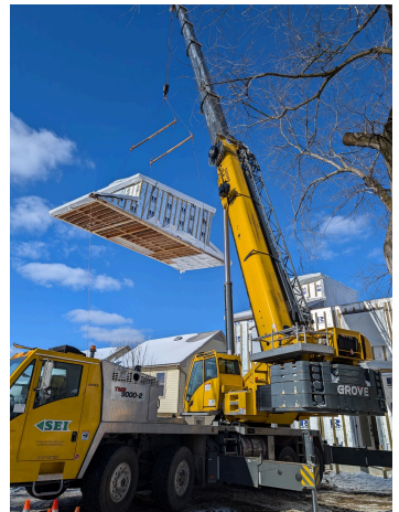
Module, a Garfield-based company, builds pre-fabricated homes that are placed on a concrete pad by a crane. Photo courtesy of Module
