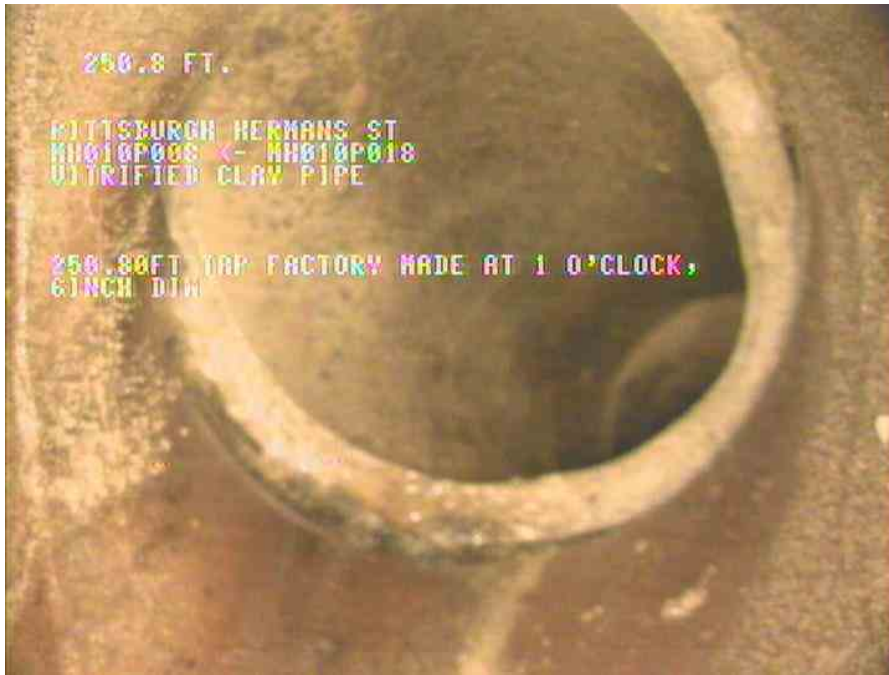
29, 00:10:30, 250.80ft Tap Factory Made at 1 o'clock, 6inch dim
