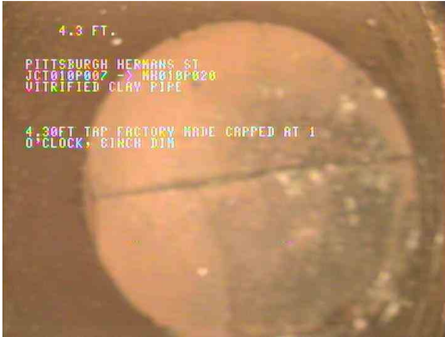
3, 00:00:57, 4.30ft Tap Factory Made Capped at 1 o'clock, 6inch dim
