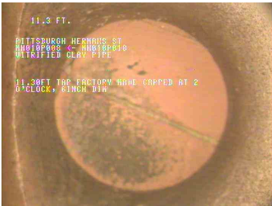
2, 00:01:10, 11.30ft Tap Factory Made Capped at 2 o'clock, 6inch dim
