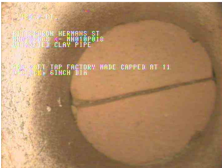
16, 00:05:09, 133.70ft Tap Factory Made Capped at 11 o'clock, 6inch dim
