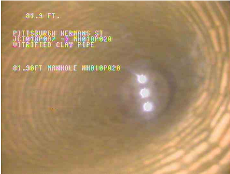
15, 00:05:14, 81.90ft Manhole / MH010P020
