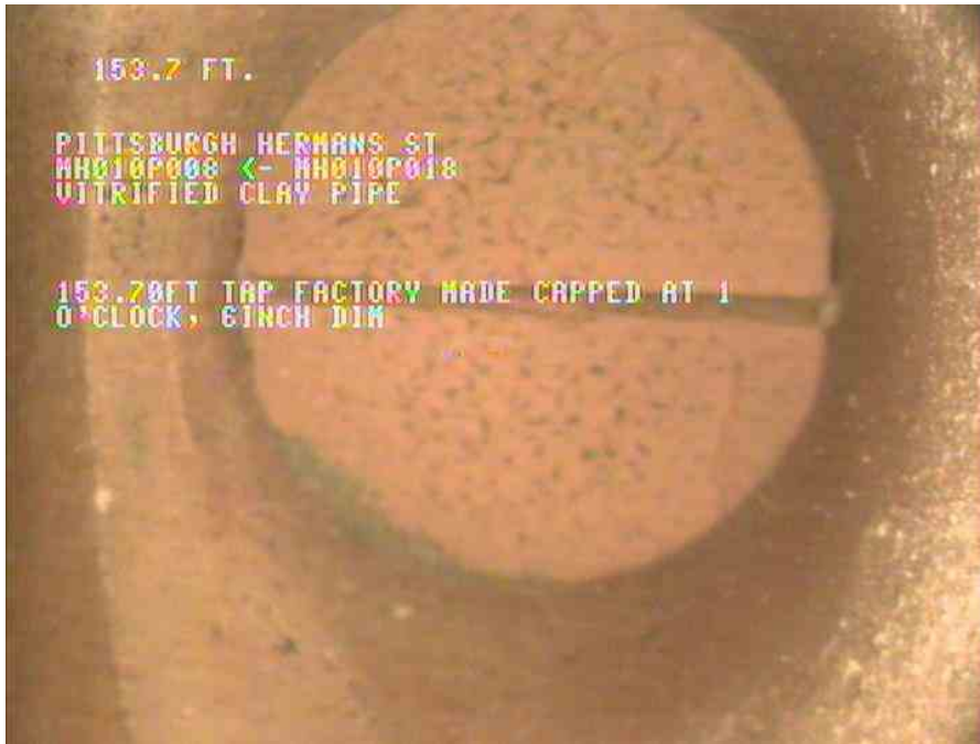
19, 00:05:57, 153.70ft Tap Factory Made Capped at 1 o'clock, 6inch dim
