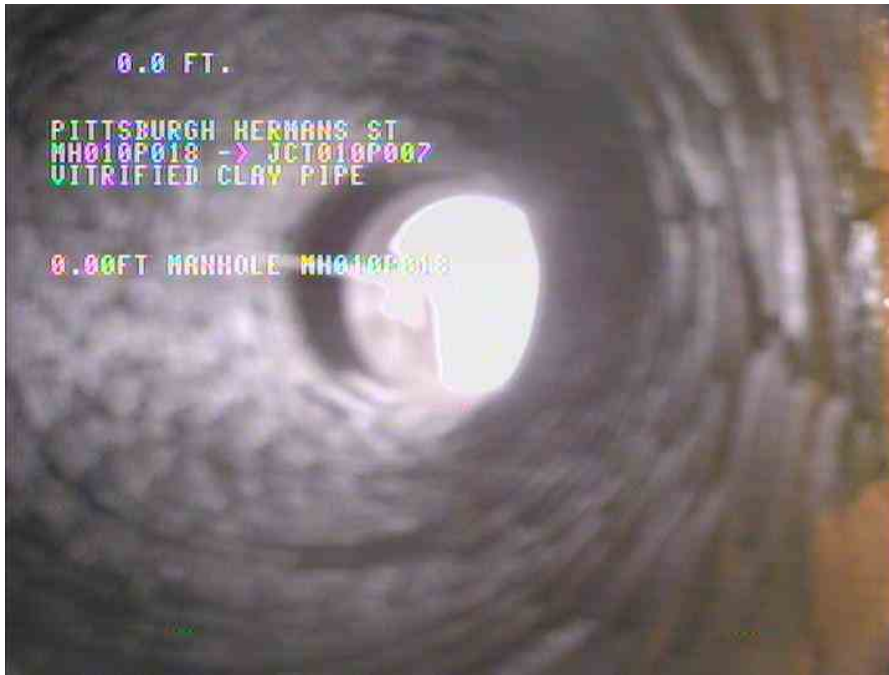
1, 00:00:00, 0.00ft Manhole / MH010P018
