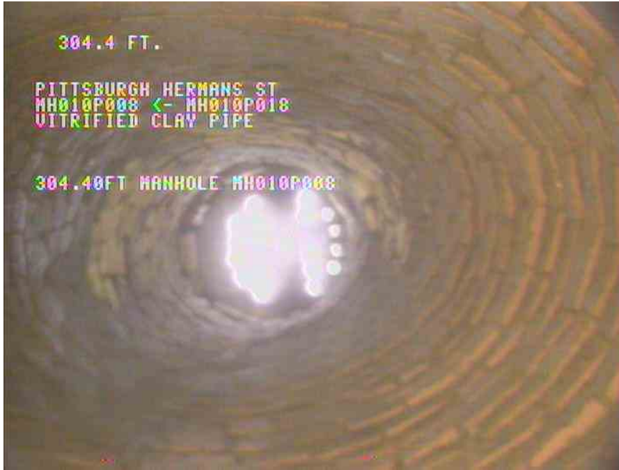
37, 00:12:46, 304.40ft Manhole / MH010P008
