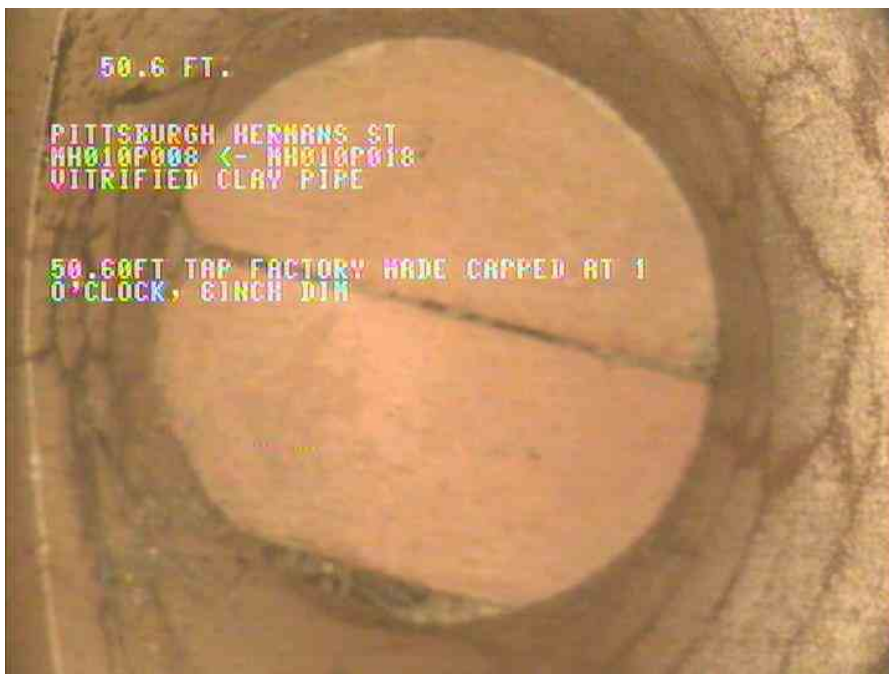
6, 00:02:21, 50.60ft Tap Factory Made Capped at 1 o'clock, 6inch dim
