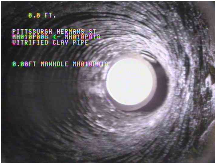
1, 00:00:00, 0.00ft Manhole / MH010P018
