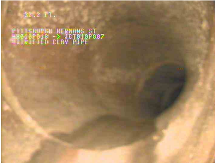
7, 00:05:55, 32.20ft Tee Connection at 3 o'clock, 15"inch vertical / JCT010P007
