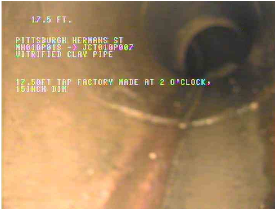
3, 00:02:42, 17.50ft Tap Factory Made at 2 o'clock, 15inch dim
