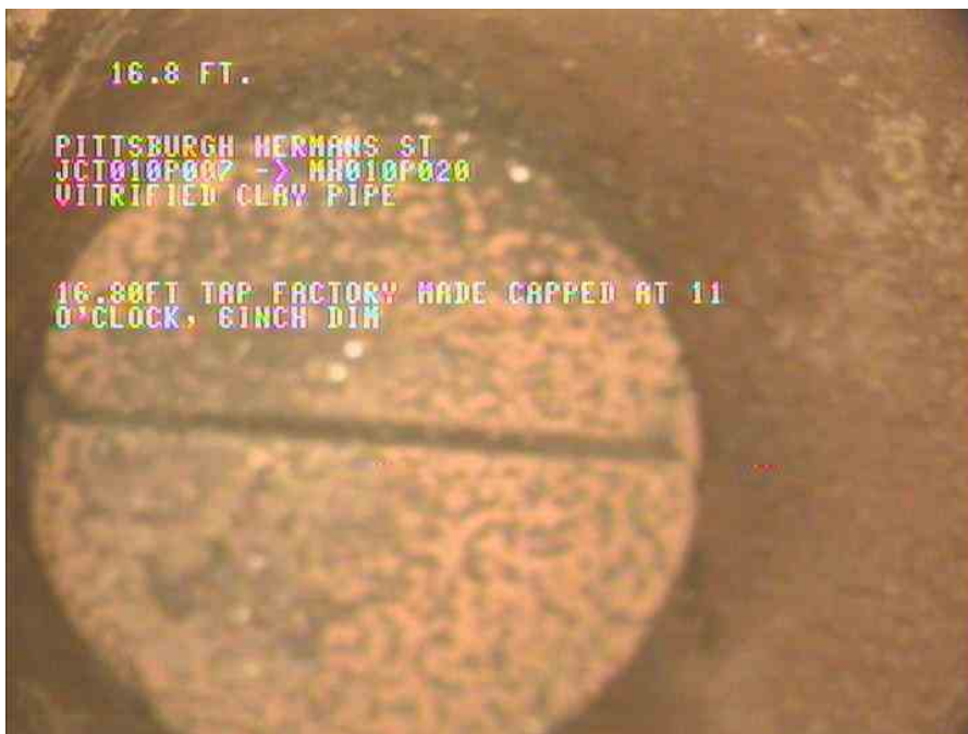
4, 00:01:25, 16.80ft Tap Factory Made Capped at 11 o'clock, 6inch dim
