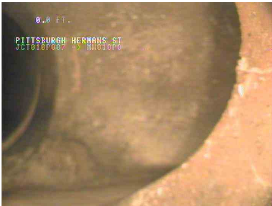
2, 00:00:00, 0.00ft Tee Connection at 3 o'clock, 15"inch vertical / JCT010P007
