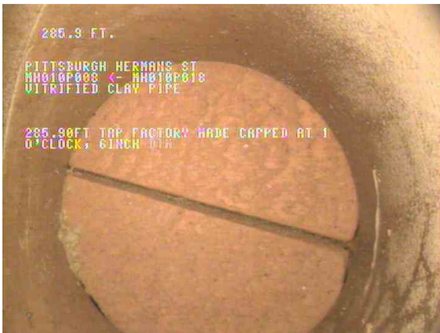
34, 00:11:50, 285.90ft Tap Factory Made Capped at 1 o'clock, 6inch dim
