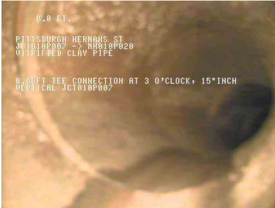
1, 00:00:00, 0.00ft Tee Connection at 3 o'clock, 15"inch vertical / JCT010P007
