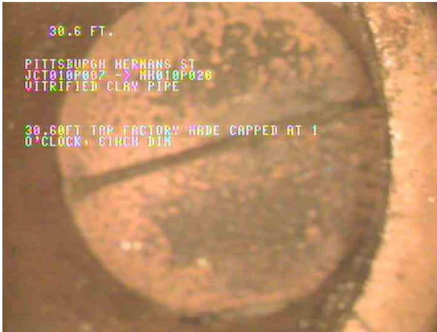
5, 00:01:54, 30.60ft Tap Factory Made Capped at 1 o'clock, 6inch dim
