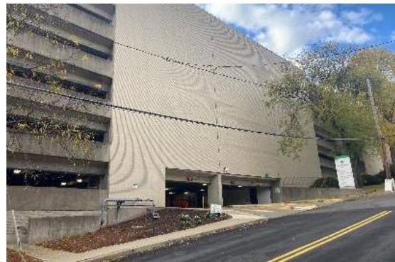
James Street Garage 9
