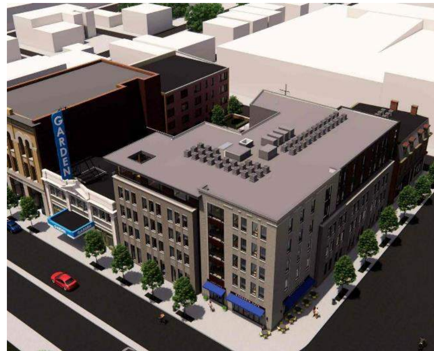
Garden Theater Block Redevelopment (Under Construction)
