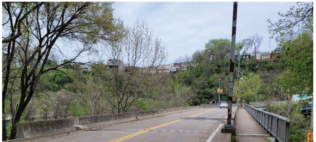
The restoration of the 30th Street River Avenue Bridge is planned, with construction expected to be complete by Fall 2023.
