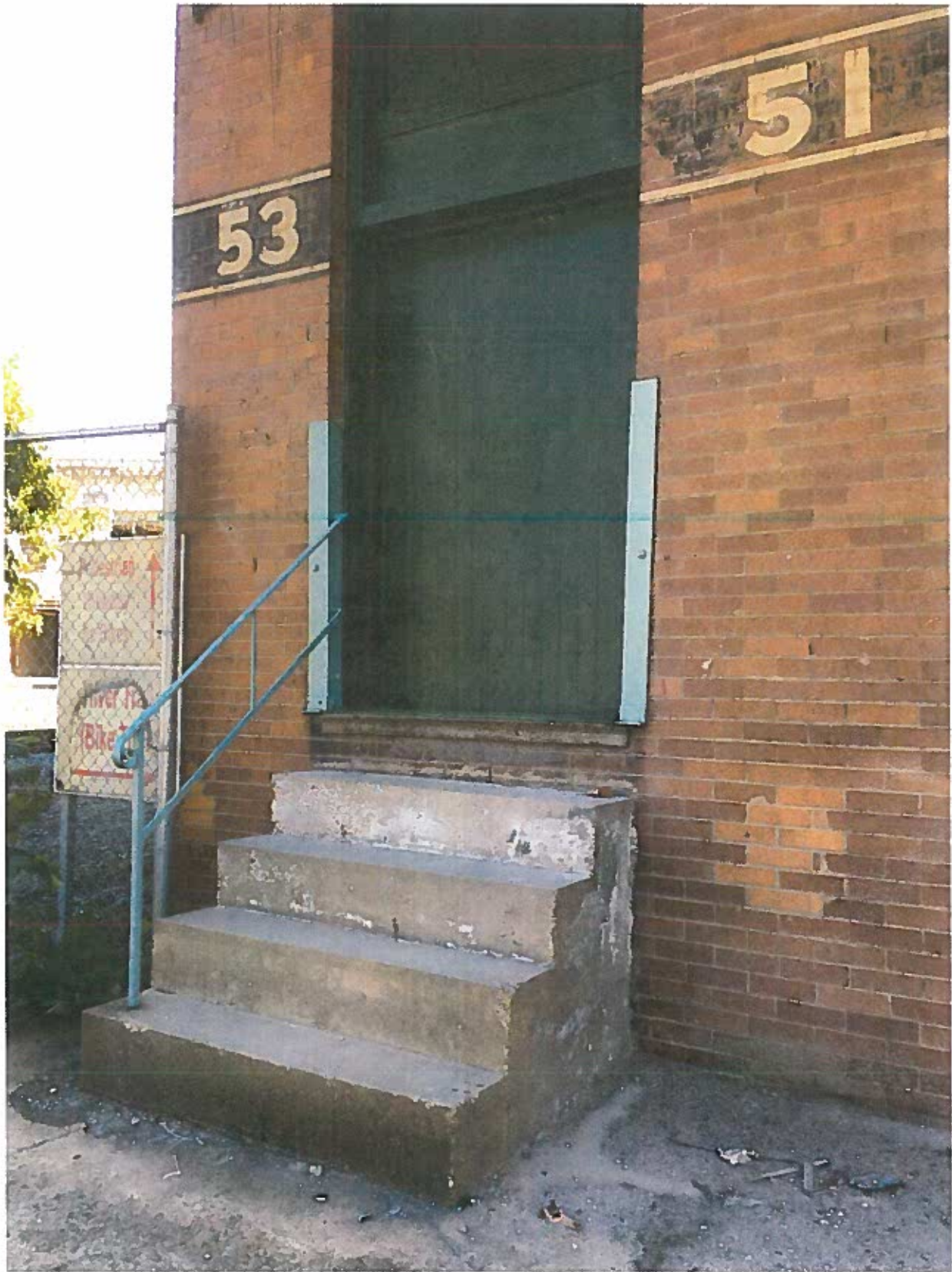
© South 3rd Street - Bay 51 - 53
