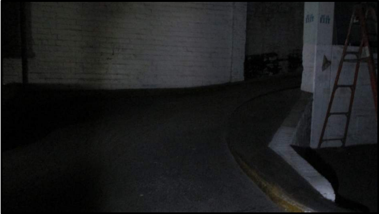
PHOTOGRAPH NO. 7 Ramp to roof looking northwest.
