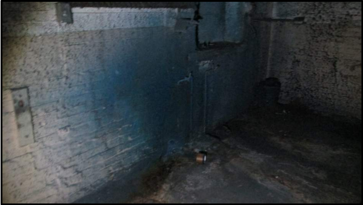
PHOTOGRAPH NO. 9 Looking northeast (second floor).
