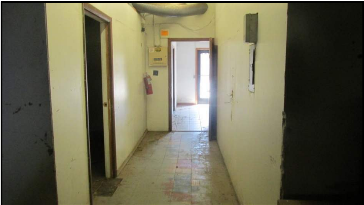
PHOTOGRAPH NO. 2 Looking south (first floor).
