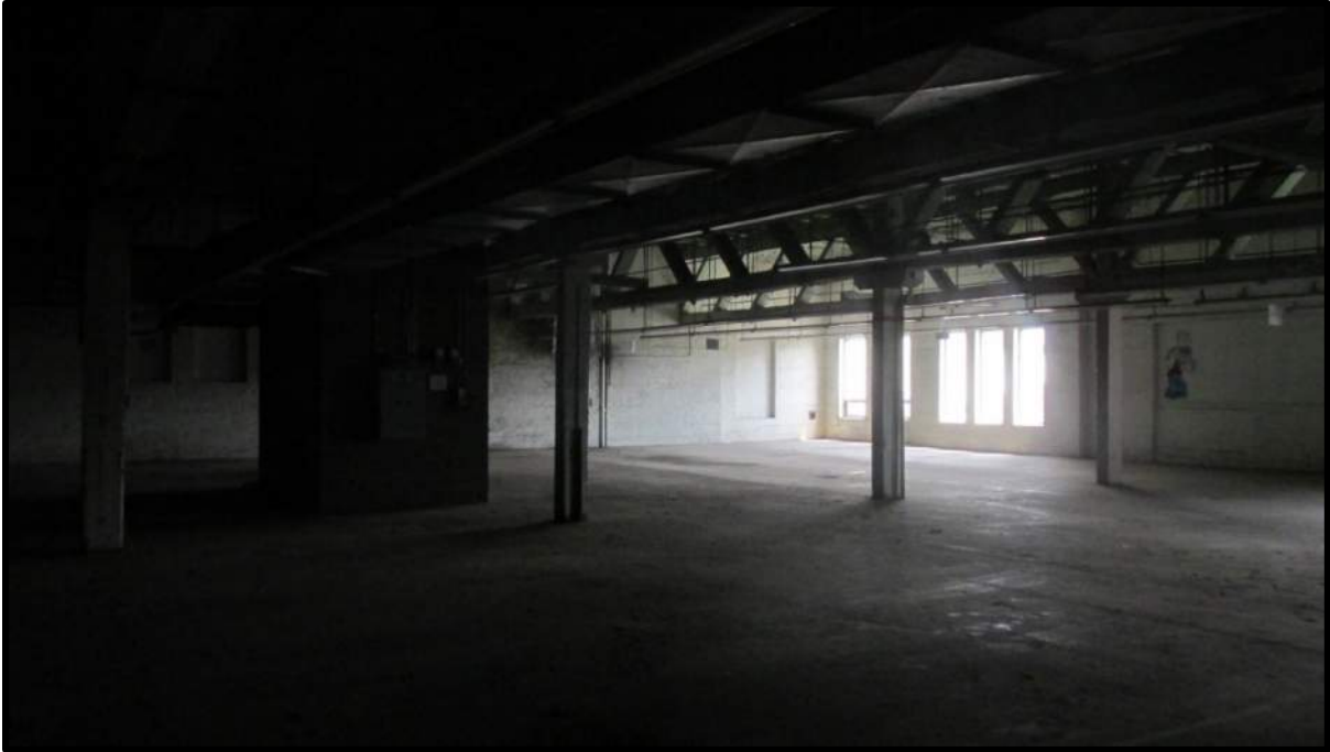
PHOTOGRAPH NO. 5 Looking south (second floor).
