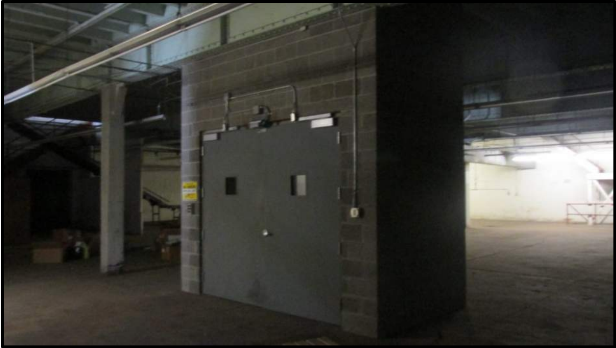
PHOTOGRAPH NO. 1 Looking northwest (first floor).
