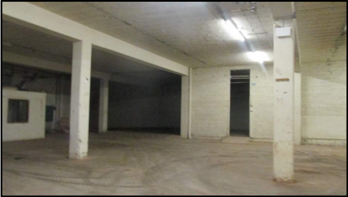
PHOTOGRAPH NO. 3 Looking southwest (first floor).
