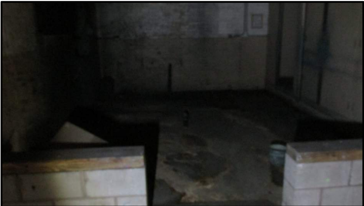
PHOTOGRAPH NO. 8 Looking south (second floor).
