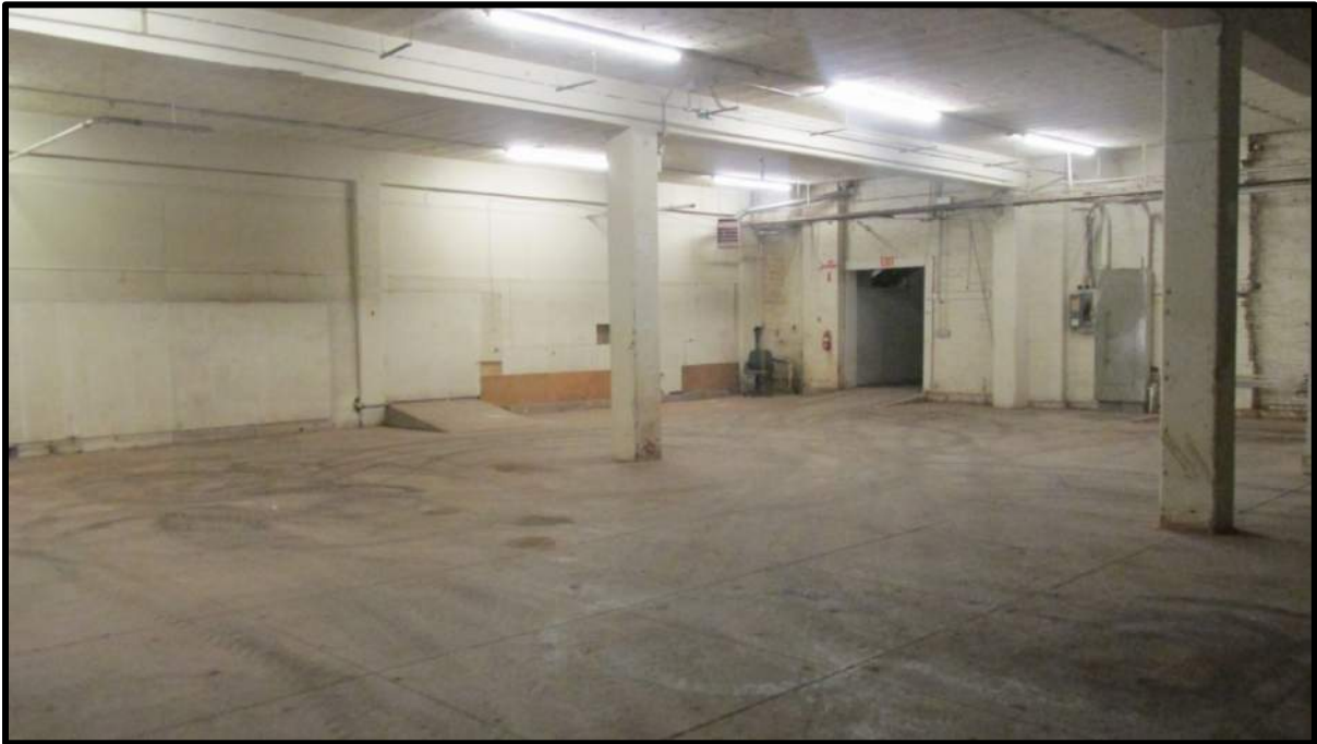
PHOTOGRAPH NO. 4 Looking northeast (first floor).
