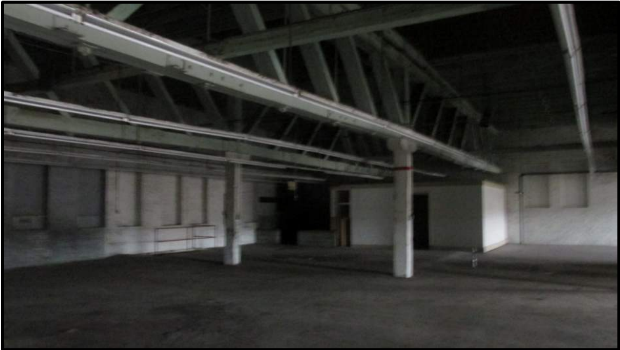
PHOTOGRAPH NO. 6 Looking northeast (second floor).
