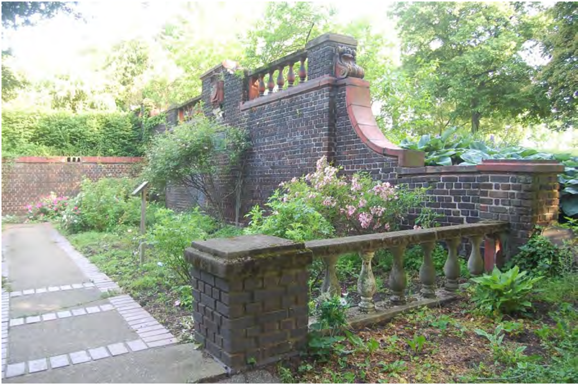
Terraced Garden, north side wall of lower terrace
