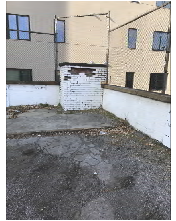
RAEBURN RD LOOKING AT BRICK STRUCTURE
