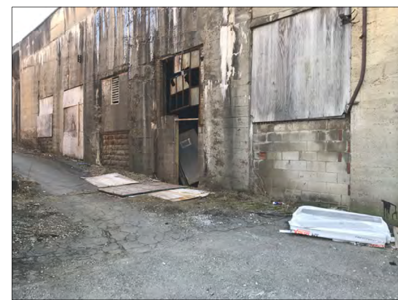
WALL BELOW RAEBURN STREET
