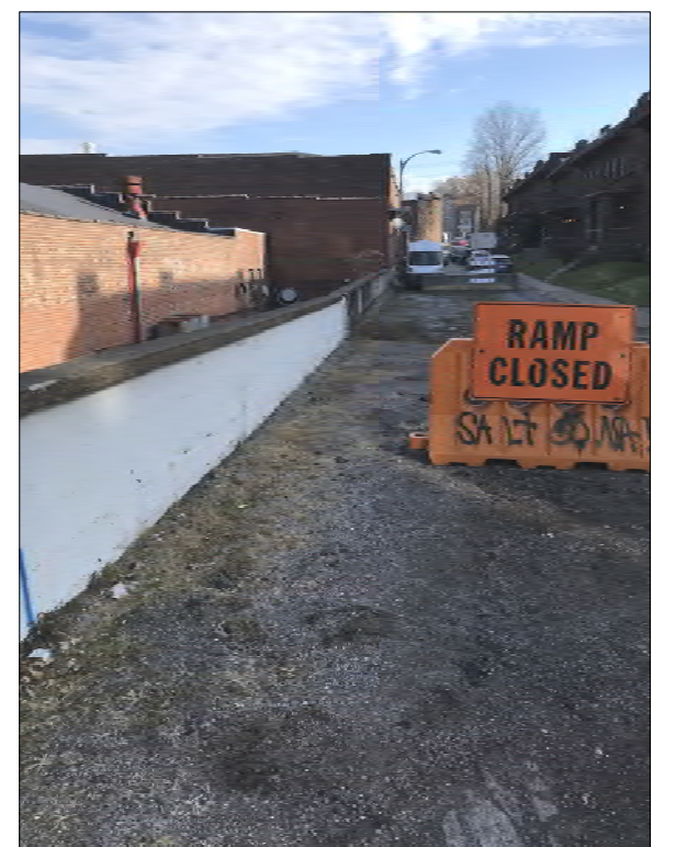
RAEBURN RD LOOKING EAST ALONG WALL
